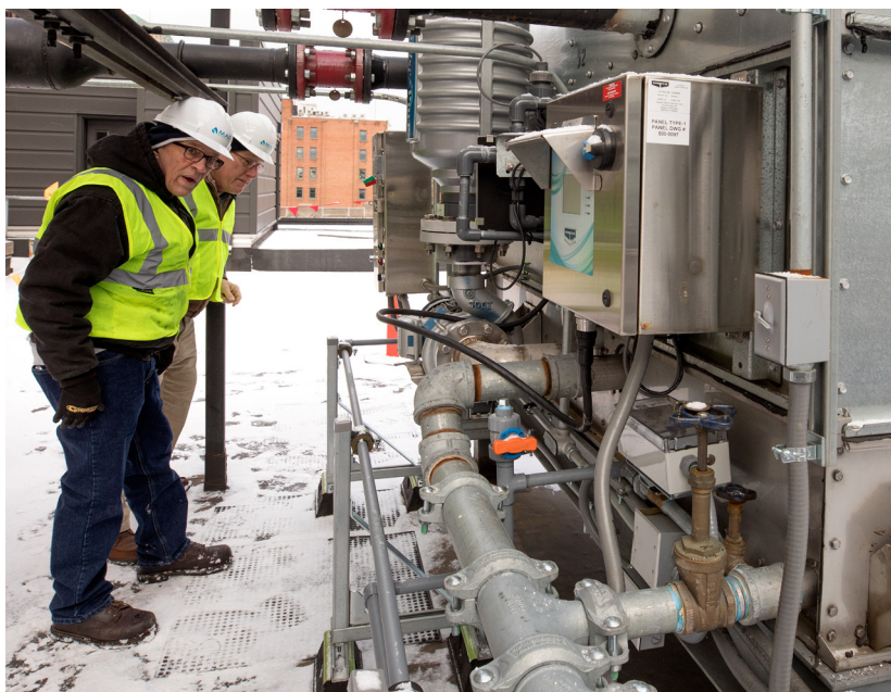
The rooftop units use an induced-draft, closed loop cooler that allowed them to be less prominent on the city skyline.
