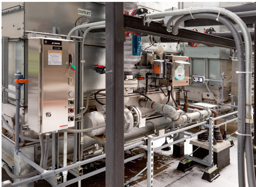
The evaporative system allowed the contractors to use only three fluid coolers.
