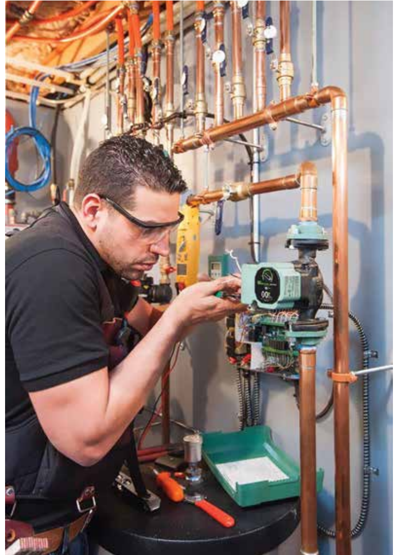
CHANGING TECHNOLOGY: The Taco 0018e allows an installer to look inside the pipes of a residential system and see what's happening from an app on their phone.
