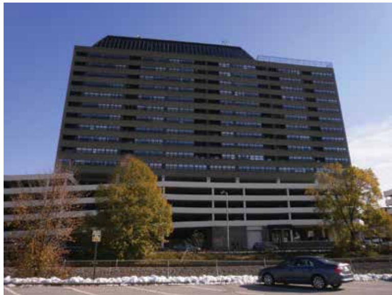
UPGRADE: Wall Street Tower, a 17-story residential facility built in 1986, recently underwent a complete HVAC retrofit.
