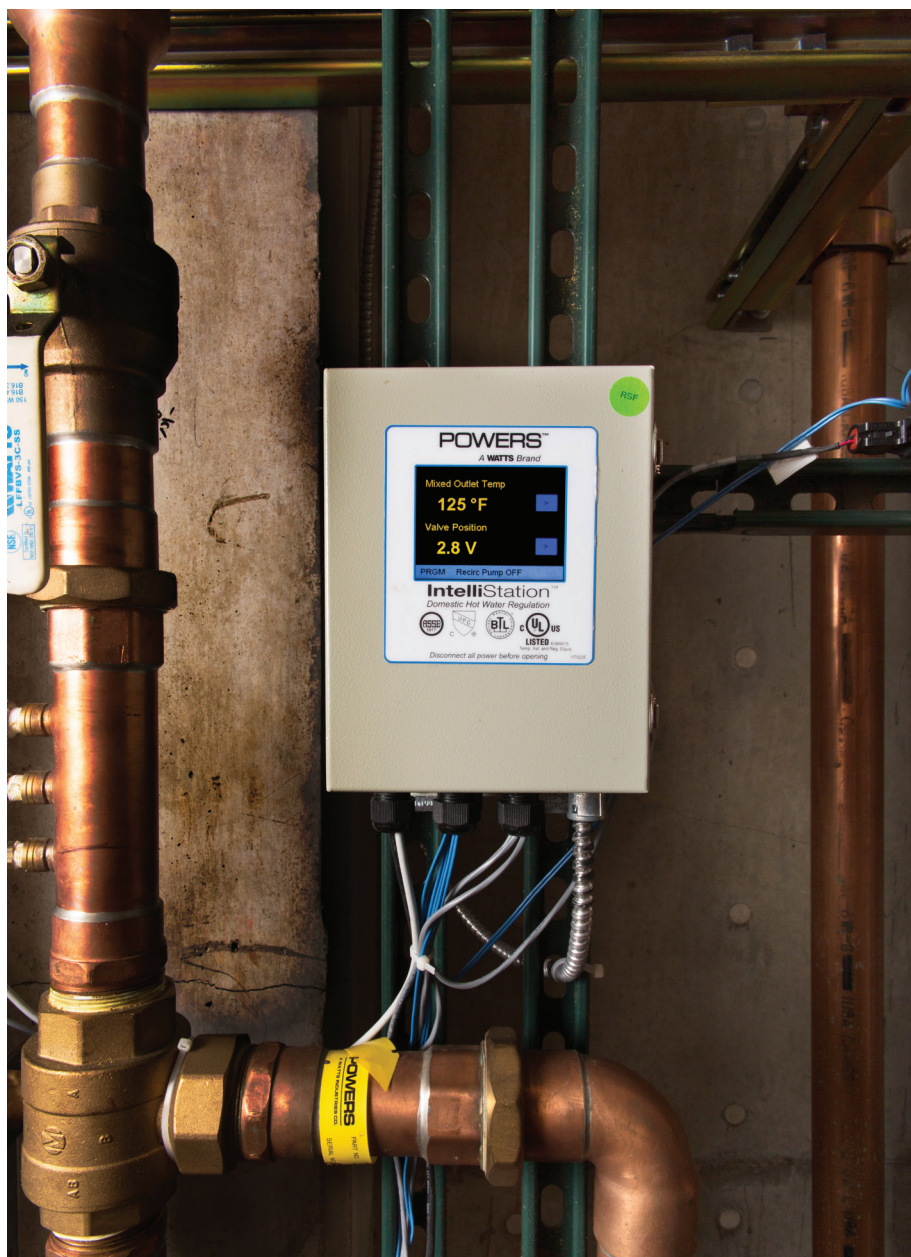
The 125-degree mixed outlet water temperature being sent through the mixed water loop to guest rooms and public restrooms, etc. (The “2.8 V” is a monitoring correlation, indicating valve position to control signal).
