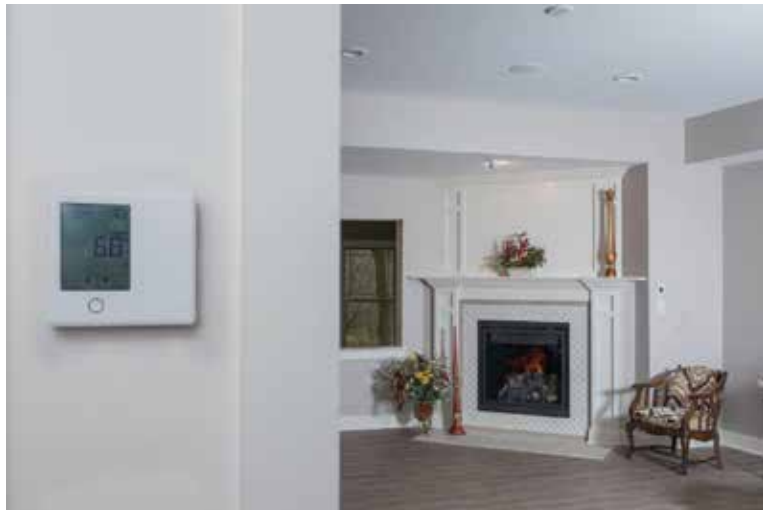
TEMPERATURE TWIST: Seven different zones allow the DeAngelis to have a warm living room, a cool bedroom, and warmer sleeping conditions for guests.
