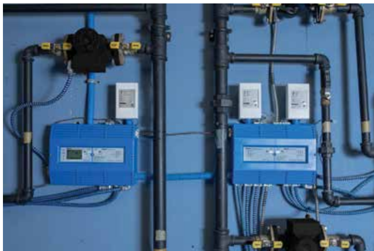
ZONING IN PLACE: The tekmar Zone Manager provides zoning solutions for two-wire tekmarNet® thermostats.
