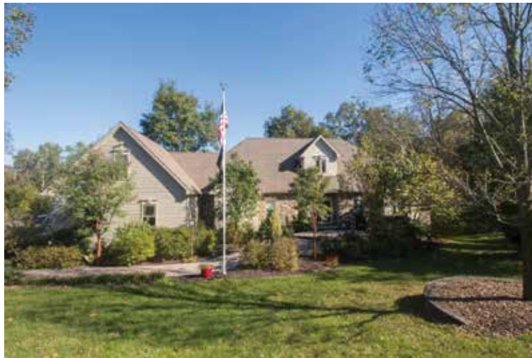
RADIANT REQUIRED: “We were determined to have hydronic heat again,” said Kathlee DeAngelis when building her Lancaster, Pennsylvania, home.
