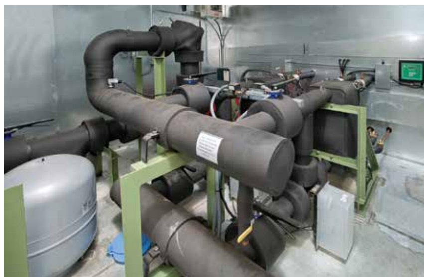
Within each Technical Systems' air-to-water heat pump is a pump house, including a variable-speed circulator and heat exchanger. TSI is a division of RAE Corp.
