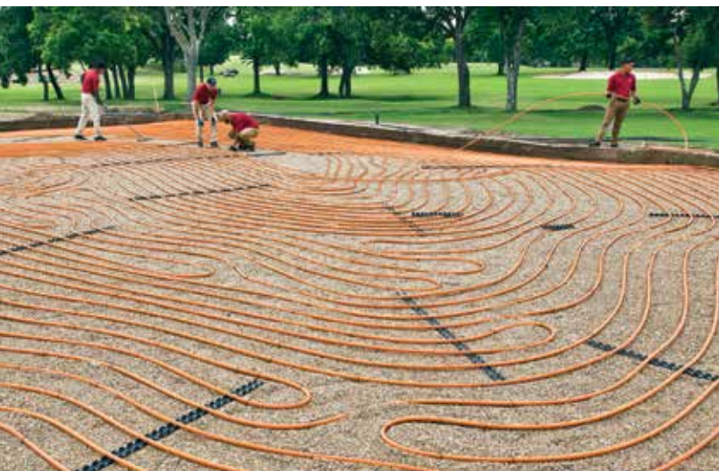
Oxygen barrier PERT tubing is laid on 9-inch centers above a 4-inch pea gravel "blanket" at Southern Hills Country Club in Tulsa, Oklahoma.
