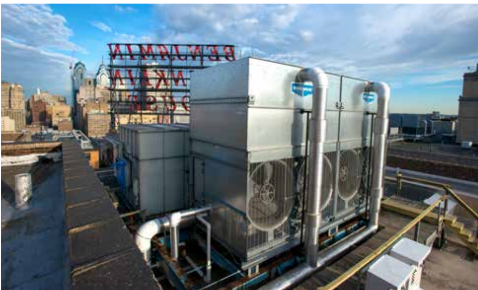
EVAPCO recreated a discontinued cooling tower to fit the tight quarters occupied by its original unit in the historic Benjamin Franklin House, simplifying the installation process for Elliott-Lewis Corporation.
