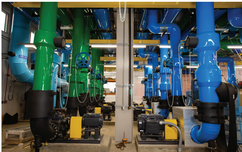
The use of plastic pipe helped reduce the amount of wastewater produced, while non-chemical treatment solutions reduced the environmental impact.
