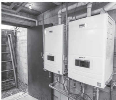
Laars Mascot FT firetube boilers are wall-hung in one of the mechanical rooms at Prairie Meadows.
