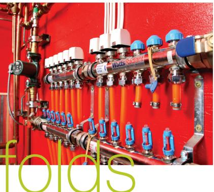
In simple terms, a manifold is the hub for central supply and return of fluids to and from a hydronic system.
