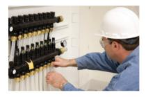
"Providing a large enough access opening to allow for tools to be easily inserted or used with the manifold is vital," he says. "If using manifolds with internal balancing valves or thermal actuators, it's important to leave enough vertical space above the manifold to allow items to be either adjusted or replaced.
