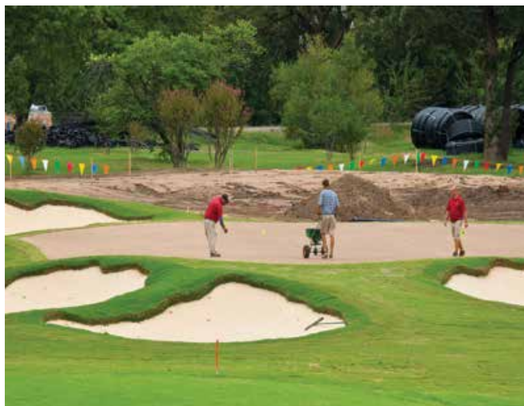
FINAL TOUCHES: After carefully prepping the green surface, Creeping Bentgrass is seeded.
