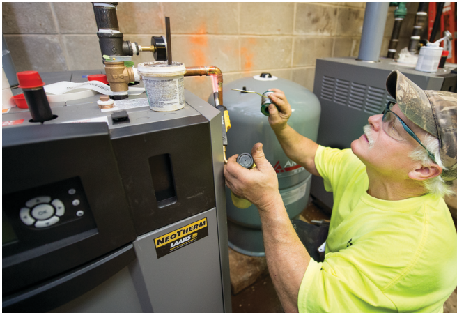
Russ Mullenberg, Faribo plumber, solders a pipe to a NeoTherm boiler's relief valve.
