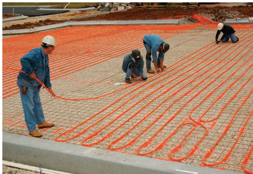
Watts Onix EPDM tubing with aluminum oxygen barrier and layers of Kevlar is resistant to jobsite abuse and UV radiation.
