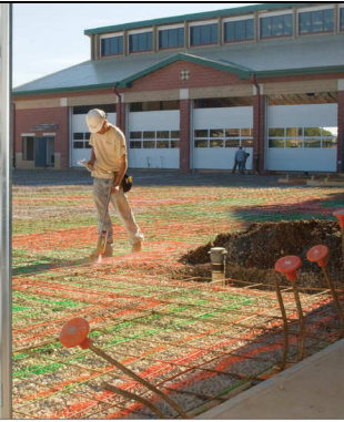
A snowmelt system being installed at a first responder station near Washington DC, just prior to tubing installation, and the concrete pour. Photo: Watts Radiant.
