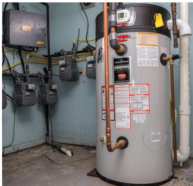
The new water heaters are the third general of Bradford White units installed since the property switched from electric to natural gas in 1990.
