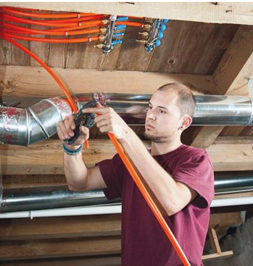
Ryan Schweitzer makes PEX connections to a radiant manifold in the home's lower level.
