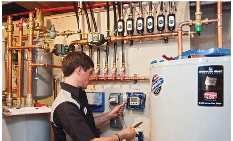
Jared Fox, Vertex lead installer, makes final connections in a central tekmar controller.
