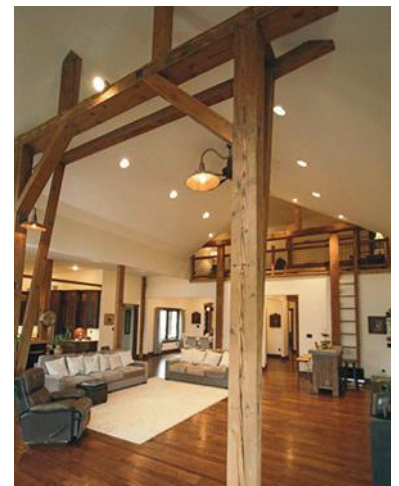
The unusual, heavy timber “strong back supports” strengthen each end of the long structure.
