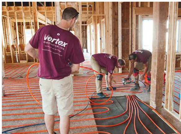
From left to right: Ryan Schweitzer, associate technician, Vince Youndt, president, and Man Khadka, Vertex Mechanical, install ½-inch Watts Radiant PEX+ tubing (walls were double-plated prior to the pour).
