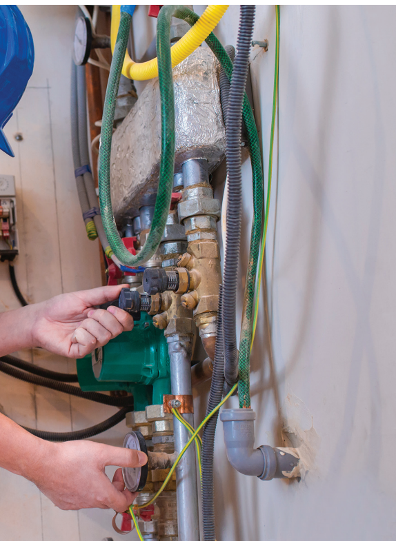
Taco's ECM wet rotor 00e VR1816 circulator offers up to 85% savings in energy consumption compared with standard circulators of the same size.
