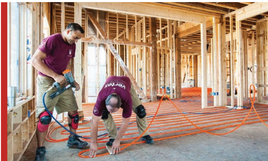
Man Khadka, installer, (left) and Vince Youndt, connect 1/2-inch Watts Radiant PEX+ tubing to the home's upstairs subfloor.
