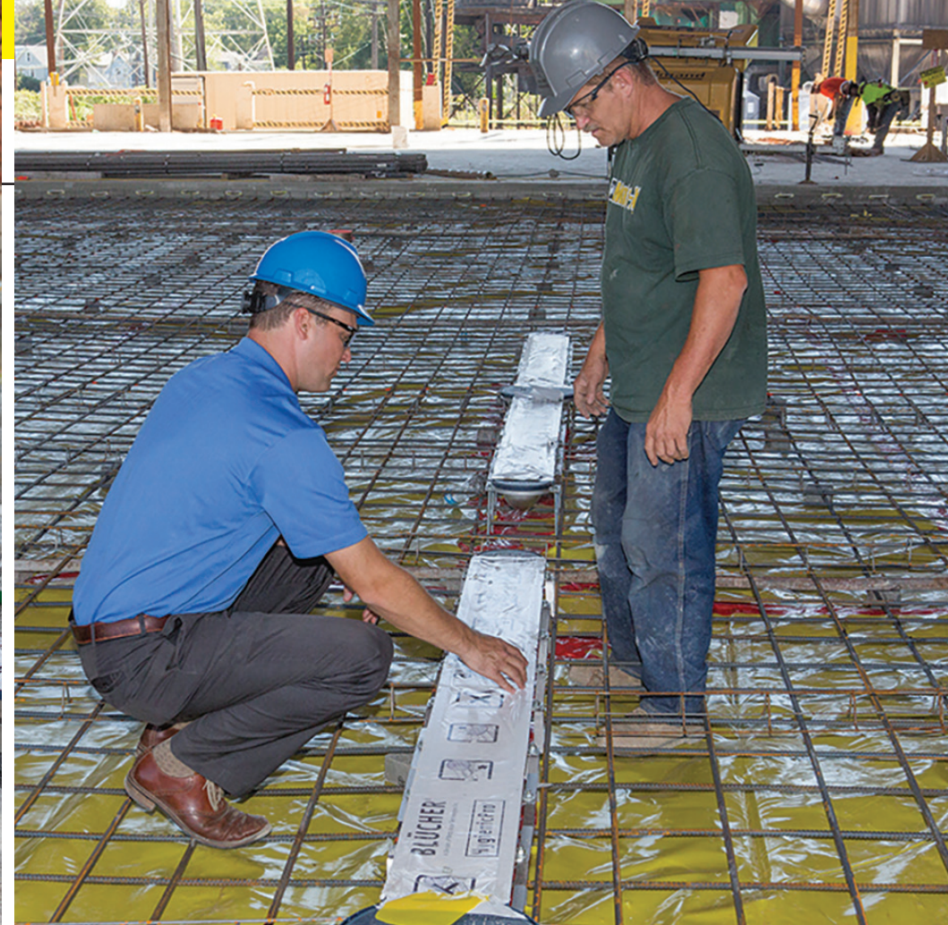
(Left to Right) Left: An AL Miller plumber installs a HygienicPro trench drain section. Right: Brett Mullins, Disney McLane salesman, left, and Denny Peace, AL Miller Plumber, inspect Blücher HygienicPro channel before the floor is poured.
