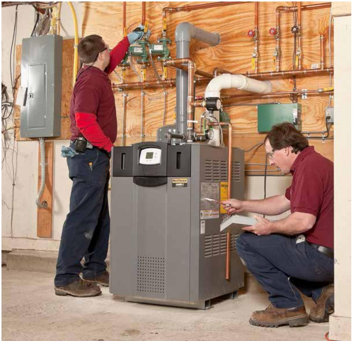
**BOILER INSTALL:** Technicians from Rymes Propane & Oil, Concord, New Hampshire, complete commissioning of a light commercial Laars NeoTherm boiler installation at Shoals Marine Laboratory on Appledore Island, New Hampshire.
