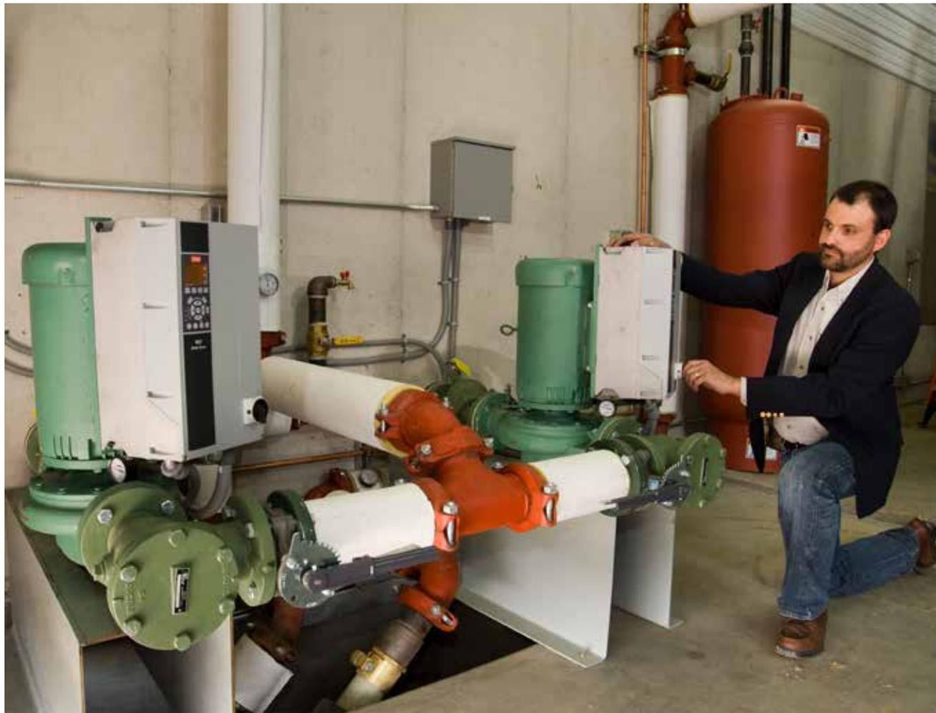
**CONSTANT CONDITIONS:** Self-sensing pumps can help improve efficiency by responding to the demands of the system and delivering a constant temperature differential across the boiler(s) at variable flows. PHOTO COURTESY OF TACO COMFORT SOLUTIONS
