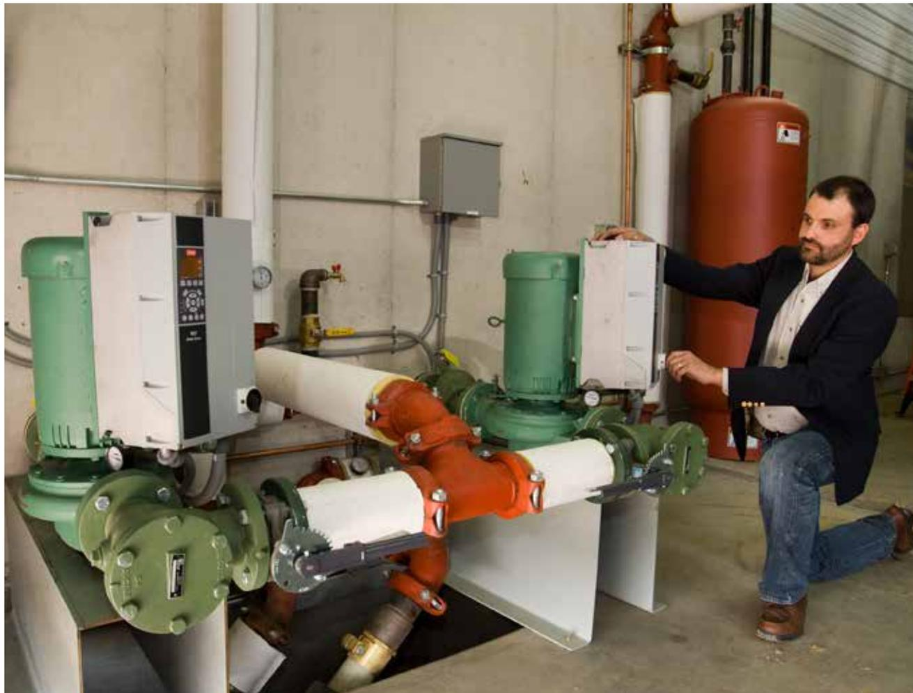
**CONSTANT CONDITIONS:** Self-sensing pumps can help improve efficiency by responding to the demands of the system and delivering a constant temperature differential across the boiler(s) at variable flows. PHOTO COURTESY OF TACO COMFORT SOLUTIONS
