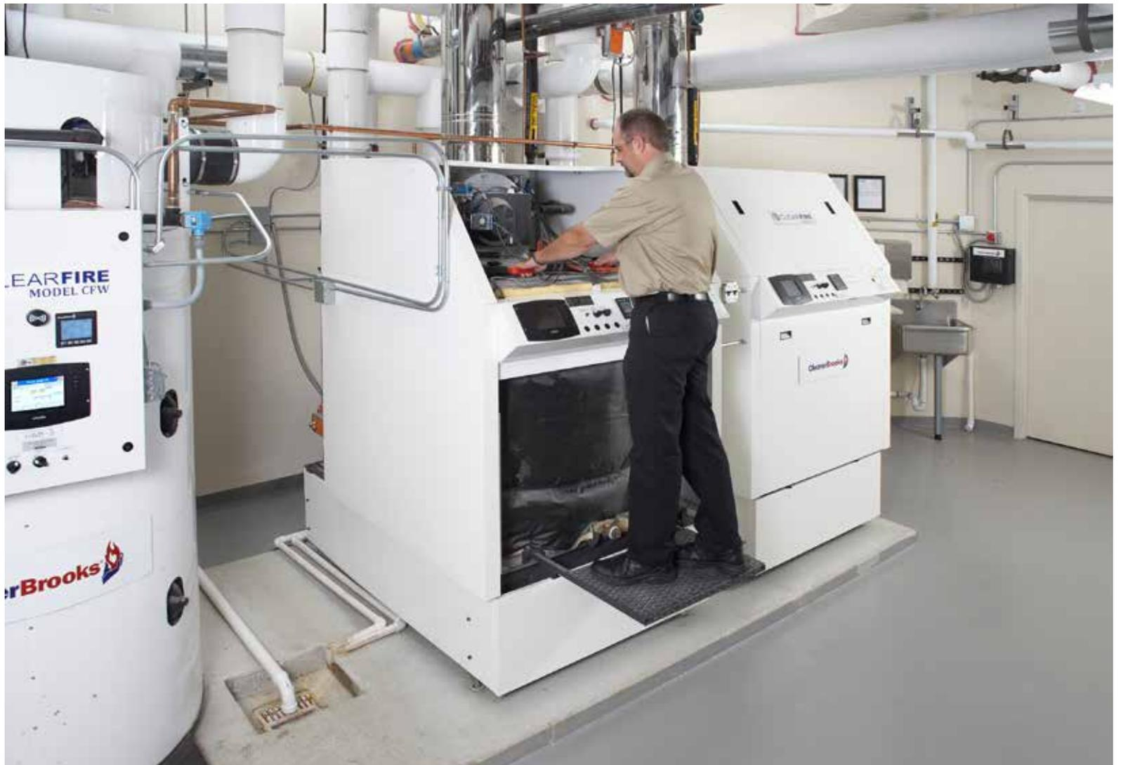
**OPTIMIZED BOILERS:** Often the simplest way to optimize energy efficiency in condensing boilers is to lower the return water temperature to the point the system is operating in condensing mode. PHOTO COURTESY OF CLEAVER BROOKS INC.
