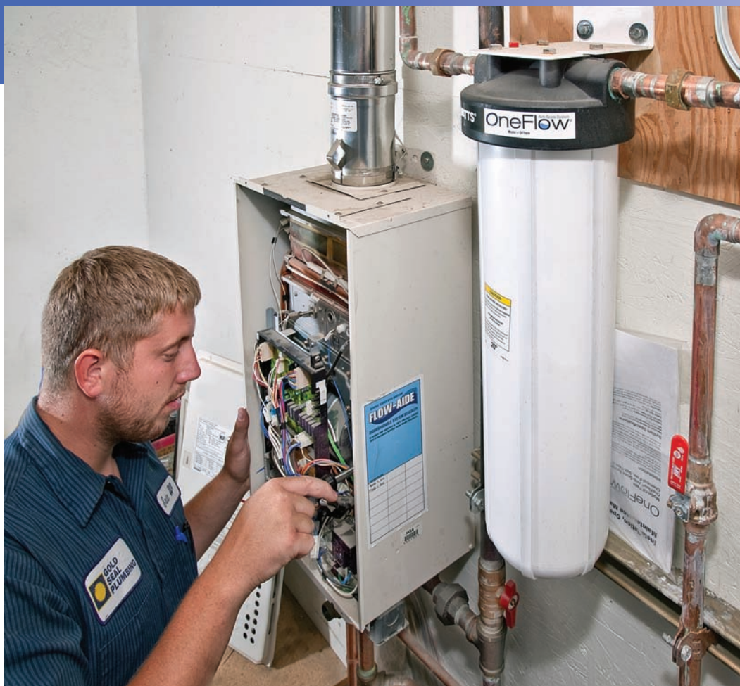
Left: A Gold Seal technician works on an instantaneous water heater. A Watts OneFlow water treatment system protects the unit's heat exchanger from mineral deposits. Dan Frisch Photography.
