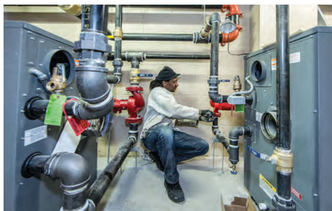
Installer Kenny White pipes the boiler injection loop.
