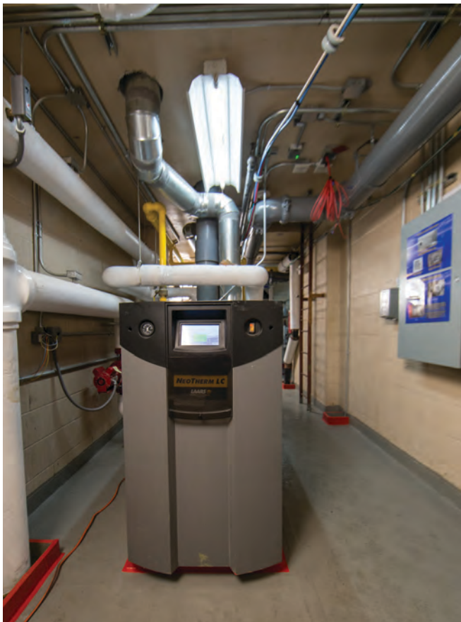
Two, high-efficiency Laars NeoTherm boilers are used to supply backup heat and cooling to the structure.
