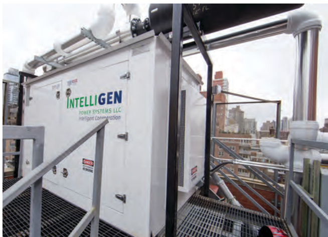
The 12-cylinder IntelliGen CHP unit is mounted on the roof of the building.
