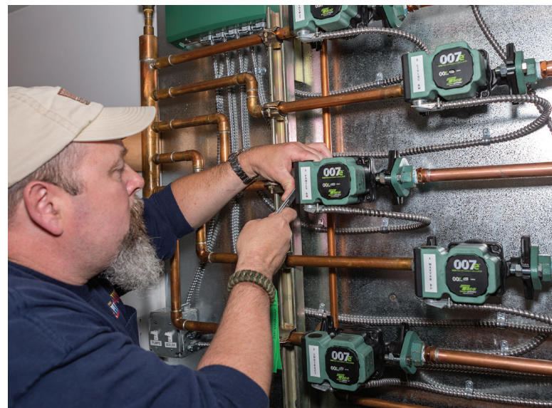
PUMPED UP: The Mallott residence utilizes four heating zones that are each pumped with a 007e, single-curve ECM circulator from Taco Comfort Solutions.
