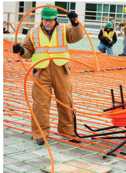
Yates feeds PEX to one Behler Crew while Behler team #2 Carl Einsig and Larry Lawrence work on other helipad PEX loops in background.
