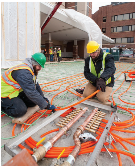
Justin D. & Ricky L. installing Watts PEX tubing in the emergency room access road
