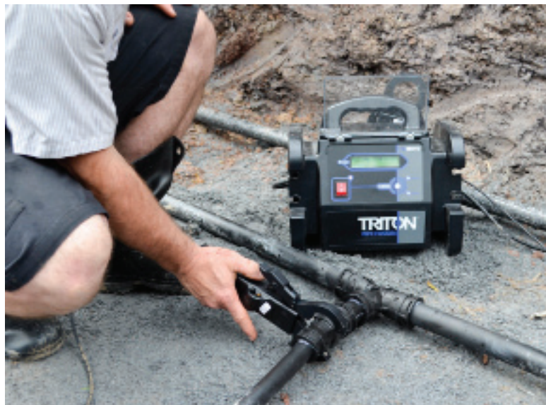
Watts' Triton HDPE pipe fusion technology
