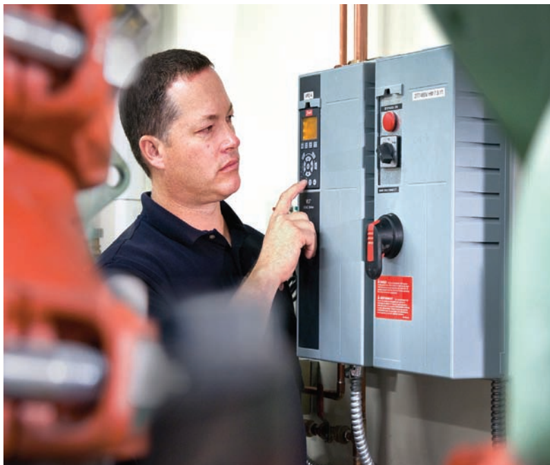
4G Project Manager, Cory Hanninen programs a VFD during commissioning. Common Ground photo.
