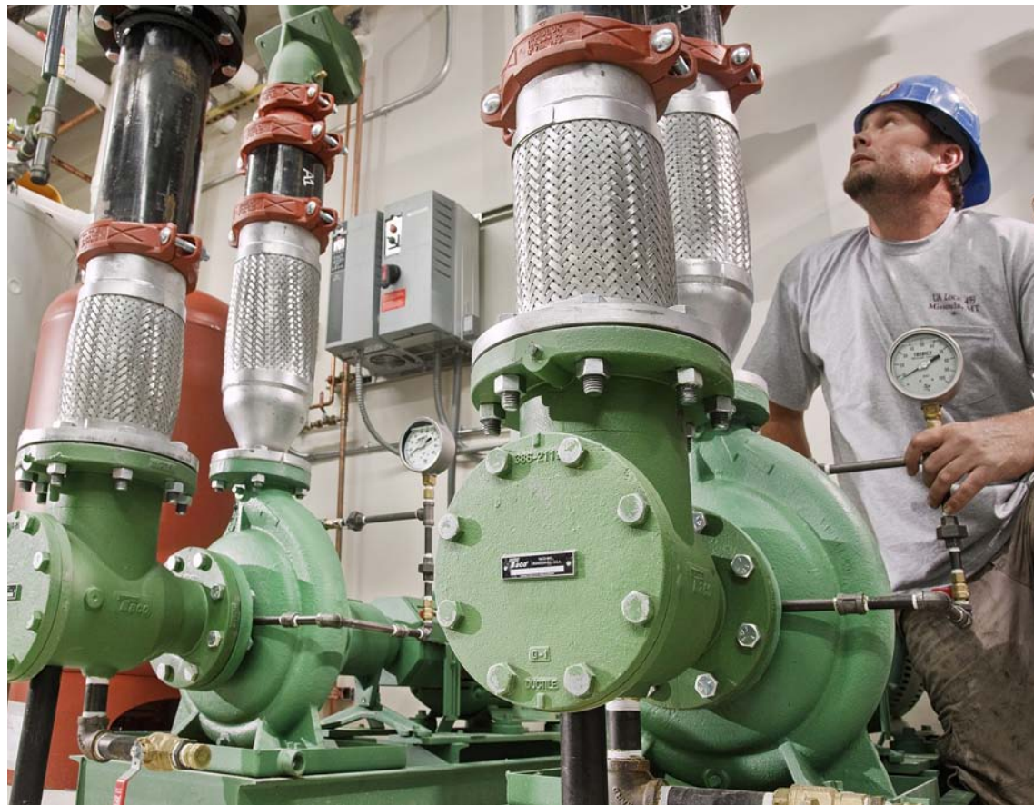
4G Project Foreman Hans Halverson works on one of four VFD-powered pumps that serve the oncology facility's heating and cooling systems. Common Ground photo
