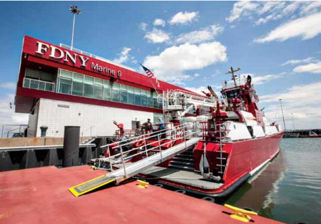
The Marine Company 9 firehouse in New York City (background) features nine solar panels with 22 evacuated tubes. The solar thermal array provides domestic hot water and space heat.
