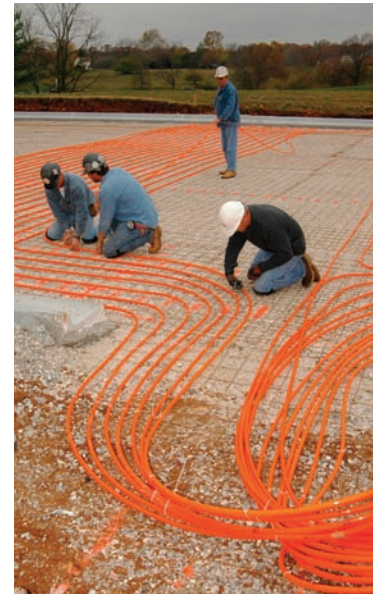
Action, Inc. installers secure 3/4-inch PEX to reinforcement wire. Watts Radiant photo by Dan Frisch.
