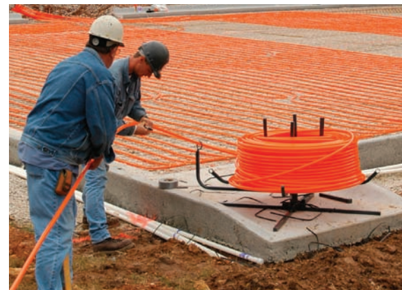
Action, Inc. installers secure 3/4-inch PEX to reinforcement wire. Watts Radiant photo by Dan Frisch.
