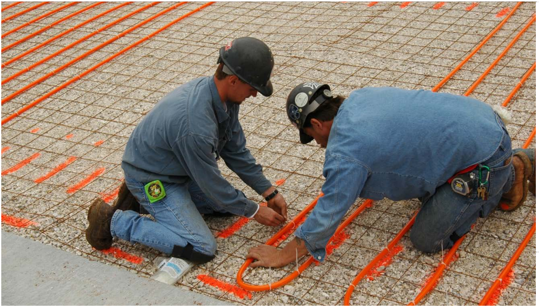
Most of the snowmelt loops were about 400 feet long; here the PEX is secured to re-wire. Watts Radiant photo by Dan Frisch.
