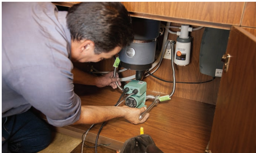
Plumber John Mohammed installs a Taco Genie hot water recirculation system.
