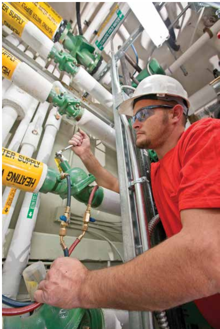
WATCHING THE WATER: Scot Walston, head service technician for Proctor Mechanical Corp., Des Moines, Iowa, adjusts the water flow through a Taco Inc. balancing valve.
