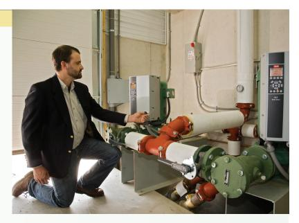
reduction in pump power. At half speed only 1/8 of the full horsepower is required. By reducing speed to a third, power is reduced to 1/27th. In addition, with variable speed, power is gradually increased. This softstart is beneficial to the motor, pump and system components. So, by reducing pump speed to match the load, energy is saved and equipment longevity is greatly improved.
