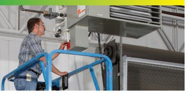
When deciding on a unit heater, you must know how much heat is needed. Information about sizing a heater and estimating monthly energy costs can be found on manufacturer websites, or by consulting with a manufacturer's rep.
