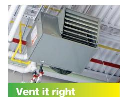
A heating system is only as good as the venting system it's connected to. A poor vent system will not only cause problems with proper combustion of the fuel being burned, but it can also lead to spillage or leakage of the products of combustion into the heated space.
