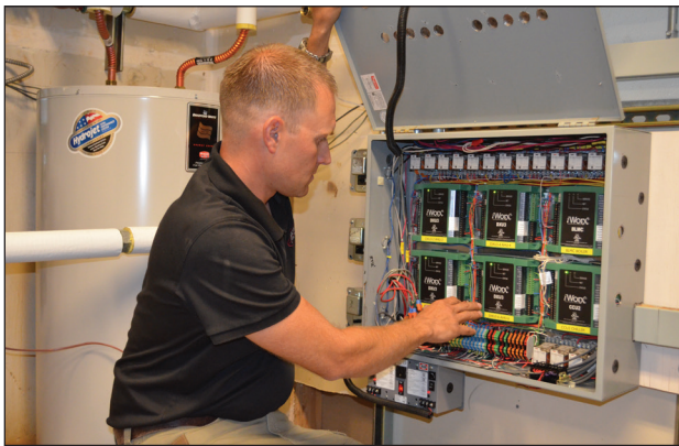
Andy Mickelson makes a final inspection of the Taco iWorX control station at First American Title Co. in Missoula, MT.
