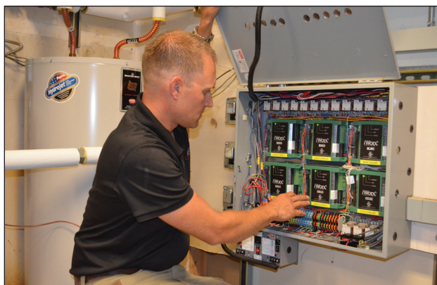
Andy Mickelson makes a final inspection of the Taco iWorX control station at First American Title Co. in Missoula, MT.
