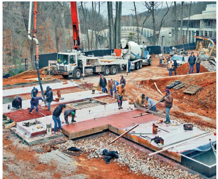
Wright had built the house on a grid system, which crews had to duplicate for the concrete pour.
