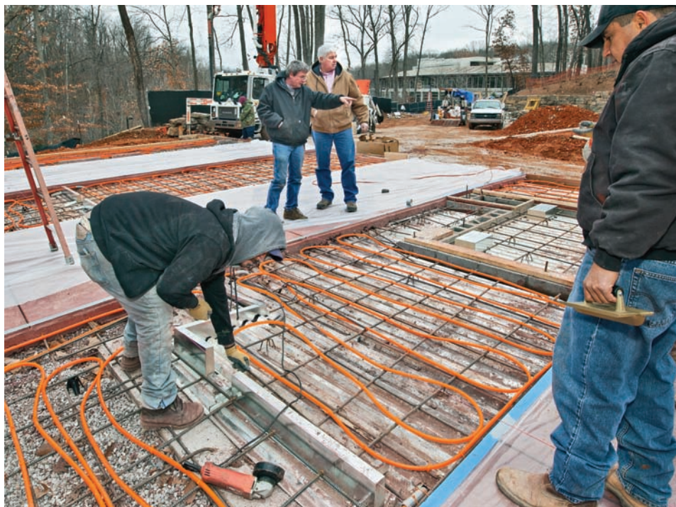
Workers first installed Watts RadiantPEX+ tubing in alternating sections, with terminations in the basement below.
