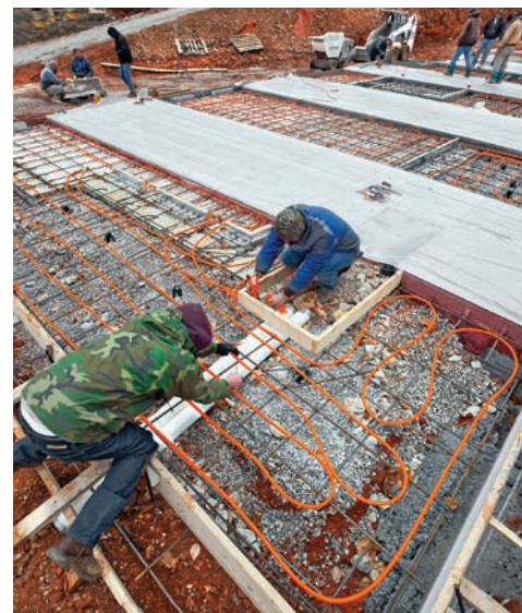
The entire structure, including the snow-melted patio outside, is radiantly heated.
