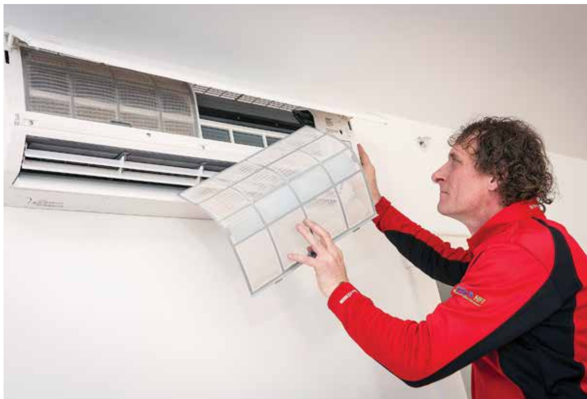
Shearer installs the indoor coil unit on one of 79 Fujitsu RLXFZ units.
