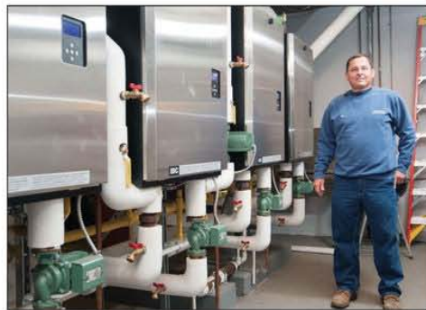
Jim Godbout "dotting i's and crossing t's" at a job site.
