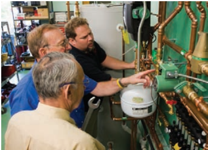
Riley (center) and Mike Muzzy, supervisor (back), show Charlie Bursey, F.W. Webb salesman (front), how a mixing valve is installed.
