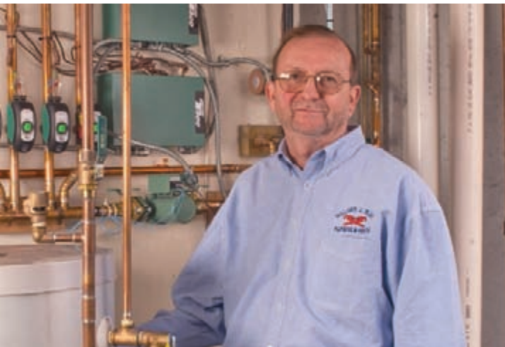
Bill Riley, owner of William J. Riley Plumbing & Heating, Warwick, R.I., is proud of a recently completed hydronics installation.
