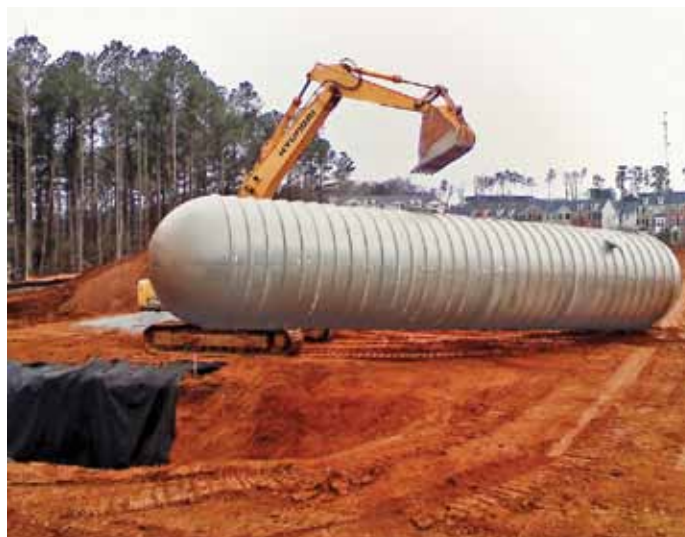
Installation of the 30,000-gal rainwater cistern that stores water for reuse for irrigation and evaporative cooling of the building's air conditioning coils
