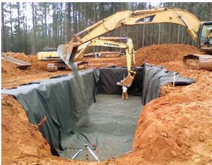
Installation of the 30,000-gal rainwater cistern that stores water for reuse for irrigation and evaporative cooling of the building's air conditioning coils
