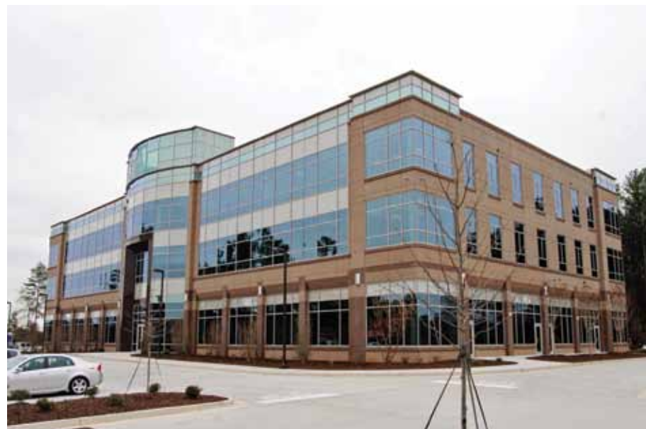
AdvancED's new global headquarters in Georgia earned LEED Gold status due in part to its rainwater harvesting and reuse system.
