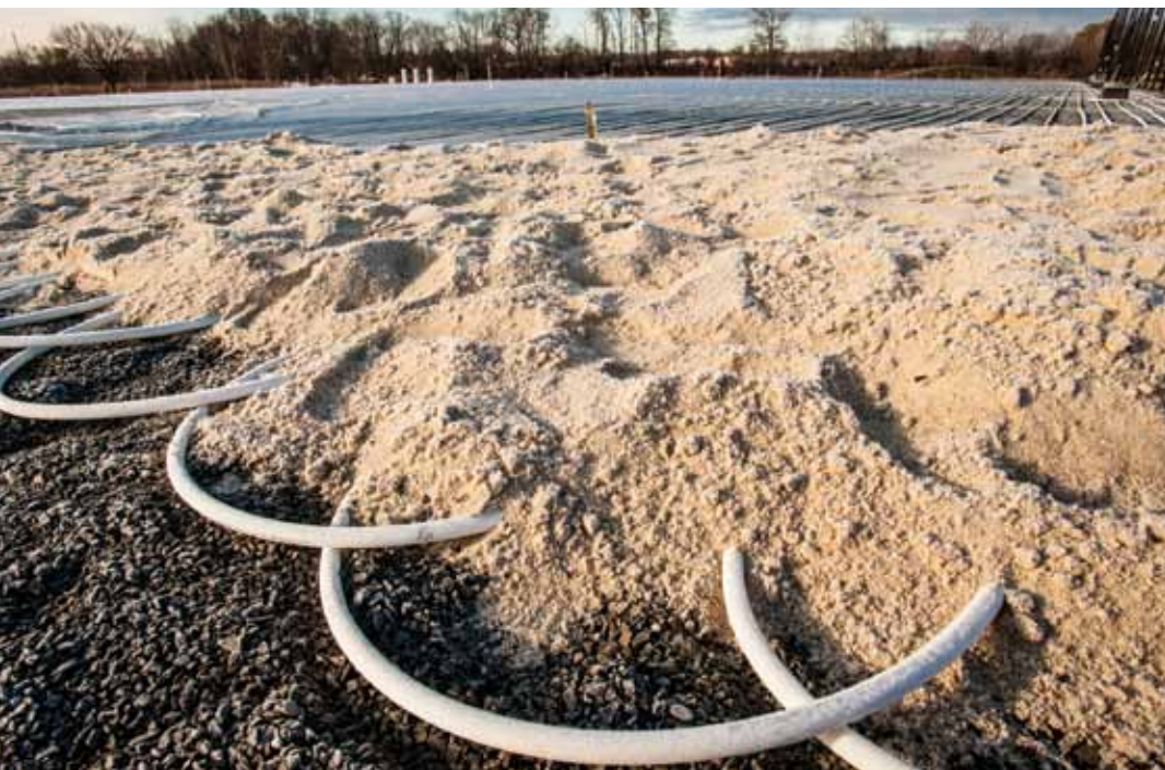
The field tubing is back-filled to hold it in place during the installation of the turf-conditioning system. The practice field has 135,300 lineal ft. of 3/4 in. Watts Radiant PEX tubing.
