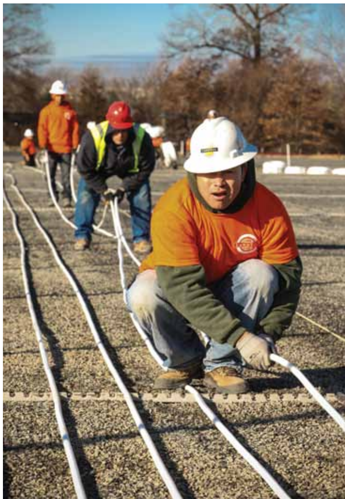
Field installers take some of the slack out of the tubing layout. Manufacturers rep firm Thermco, which designed the reverse-return layout, sized the field at 8 million Btu.
