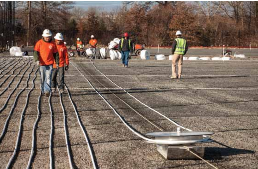
The radiant tubing layout of the New York Red Bulls' new turf-conditioned soccer practice field is accomplished with a motorized sled, developed by Althoff Industries, to keep PEX tube spacing uniform.
