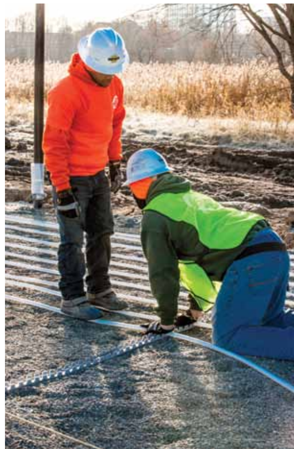
LandTek technicians install PEX tubing in the rail system — which is spiked into the stone layer — to keep it evenly spaced.
