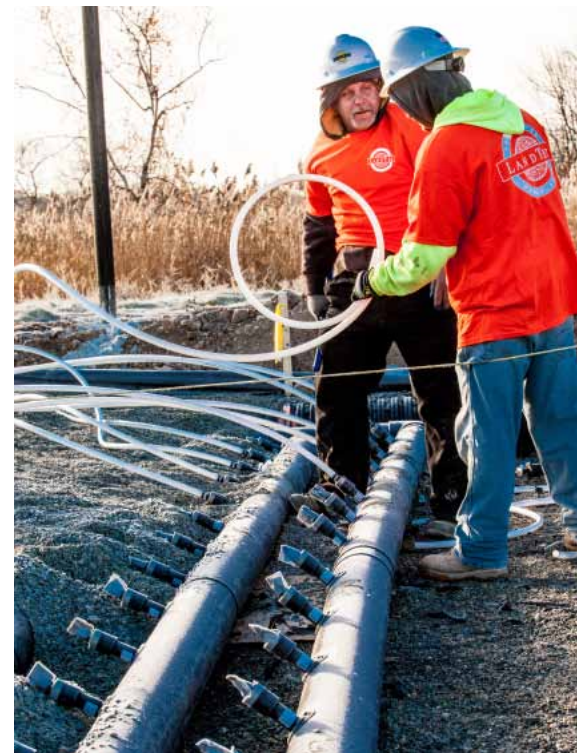
LandTek Group field personnel make tubing connections to headers at one end of the practice field. More than 50 20-ft. manifolds were heat-fused together to field-fabricate the large manifolds needed.
