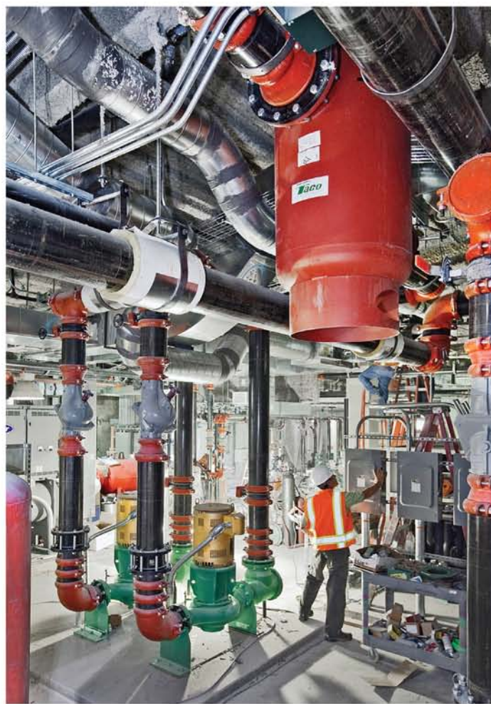
LEFT: Gary Solberg, project supervisor and manager for McClintock & Turk, Inc., assembles piping connected to a below-grade sump pump.
