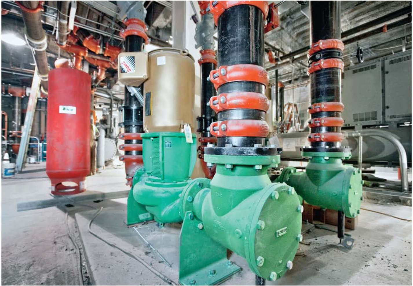
Chilled water pumps in the basement mechanical room.
