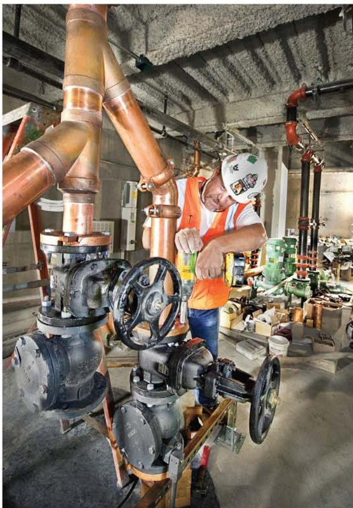
LEFT: Gary Solberg, project supervisor and manager for McClintock & Turk, Inc., assembles piping connected to a below-grade sump pump.
