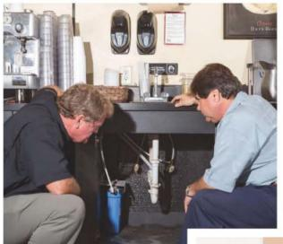
valves, etc. Limited maintenance is required; systems require media replacement every three years.
