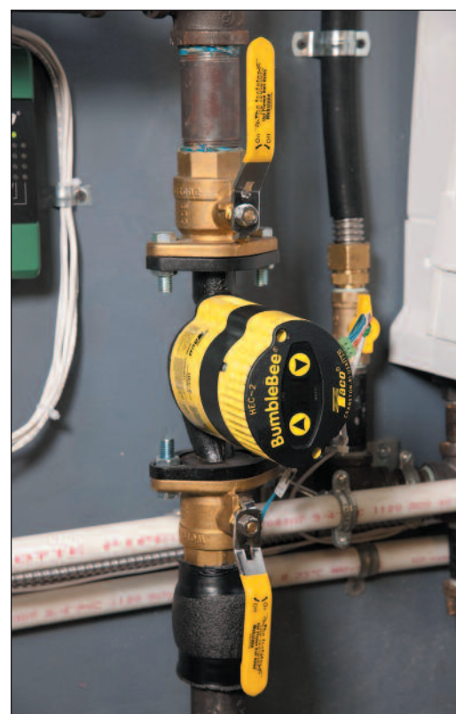
Taco's bright yellow ECM circulator, the Bumble Bee, points the system toward 20-degree delta-T operation.
