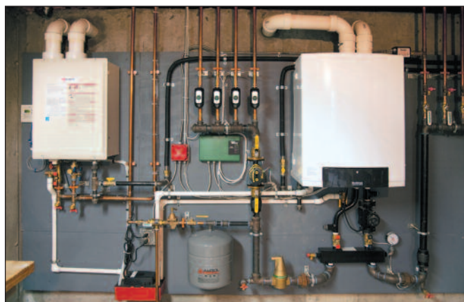
A 30 MBH, 95% AFUE, LP-fired wall-hung mod-con boiler, a Noritz tankless water heater and Taco components complete the system.
