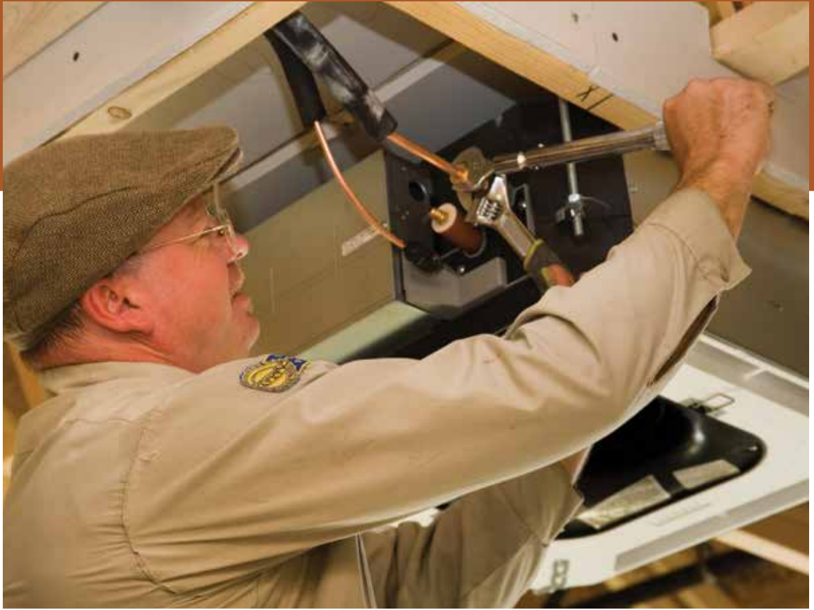
» Scott McGuire connects refrigerant lines to a Fujitsu ceiling cassette unit.
