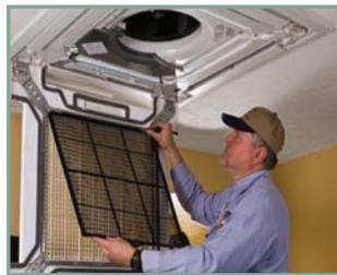
**Getting inverted** A key contributor to ductless system energy efficiency has been the introduction of “inverter” technology. Though this technology has been in use for more than a decade in Eastern and European countries, it’s a relatively new player in the HVAC sector in Canada. The inverter converts AC power to DC and uses pulse-width modulation to produce variable frequency AC current, modulating the speed of the motor to match the heating or cooling needs of the space being conditioned.
