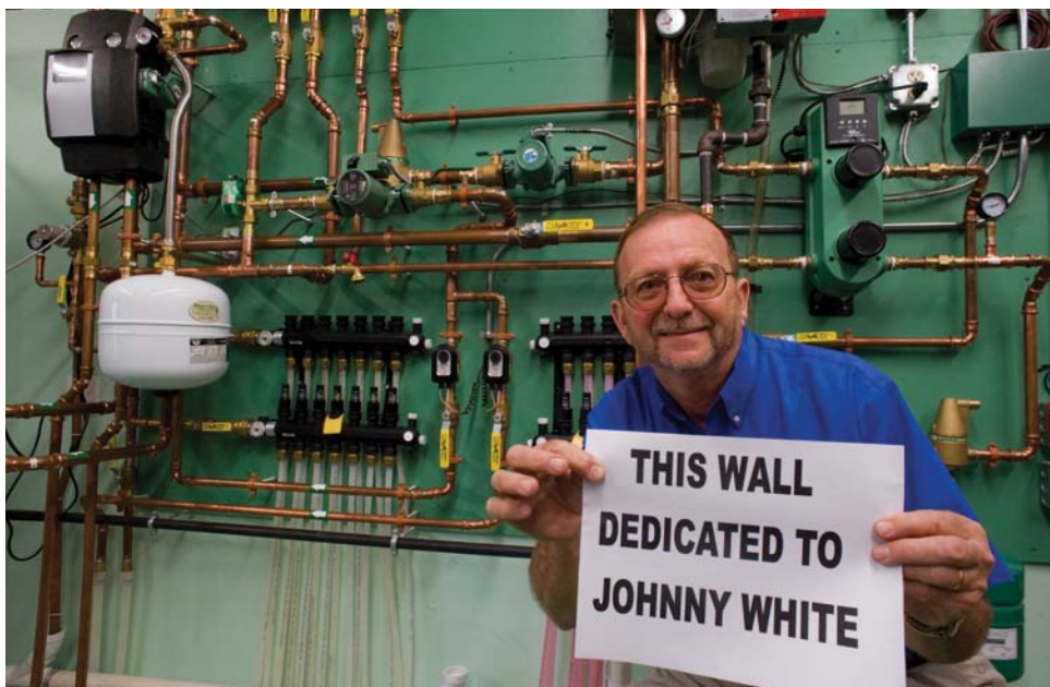
Some installing contractors just can't hide their enthusiasm for Taco.
