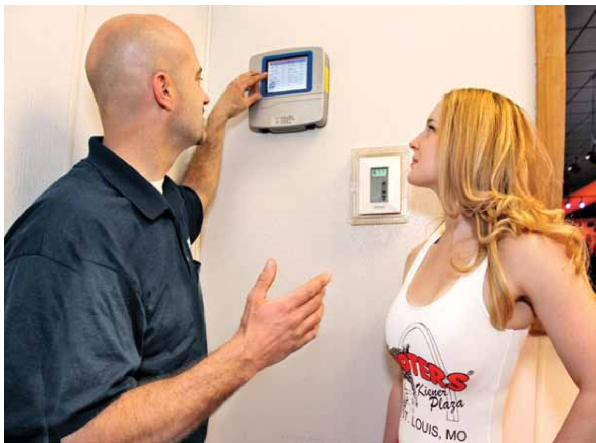
Durbin explains the simplicity of the iWorx LCI2 (local control interface) with waitress Rebecca Hern.
