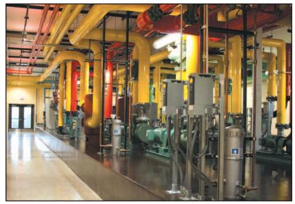
Color-coded pipe insulation allows visitors to follow system flow and operation. Each color has different meanings, specific to the loop it's part of. Red is specific to the heating loop, while dark blue identifies chilled water. ITEC's mechanical system includes six different colors.
