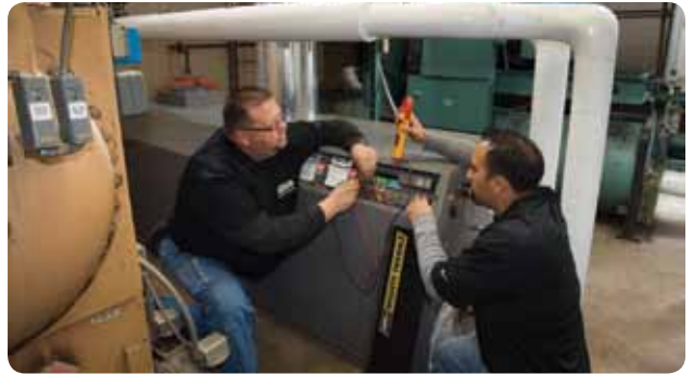
Gary Holbrook and Eric Tafoya service a Laars boiler at Summit Apartments.
