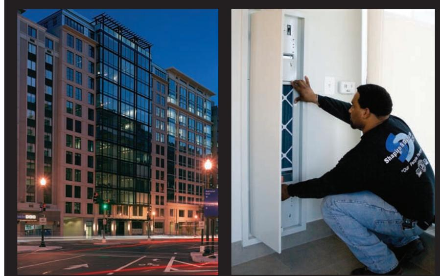
**The Alta at Thomas Circle is the first LEED-certified condo/mixed-use development in Washington D.C. Vertically stacked heat pumps in each unit were one of the first changes to turn the project green in mid-construction.**
