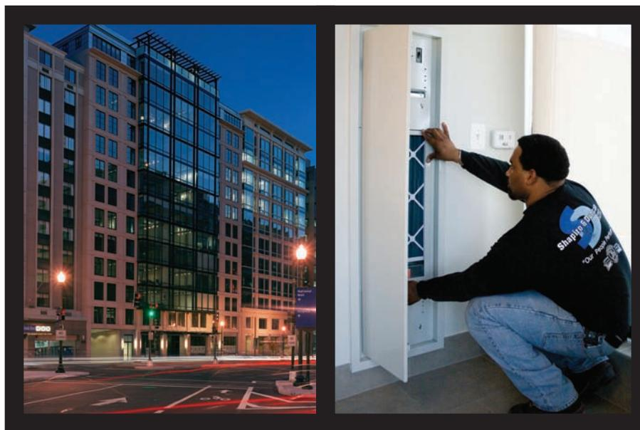
**The Alta at Thomas Circle is the first LEED-certified condo/mixed-use development in Washington D.C. Vertically stacked heat pumps in each unit were one of the first changes to turn the project green in mid-construction.**
