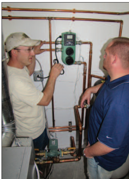
Joel Ballek shows a homeowner how to use the new Taco radiant mixing block at Stilmeyer Estates, North Pole, Alaska.
